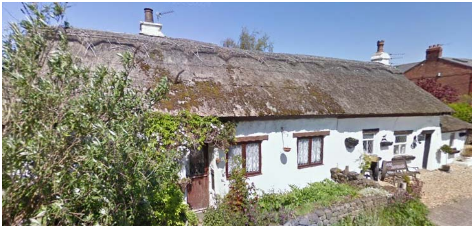
Photograph of the listed cottages at 1 & 2 Fishers Lane.
